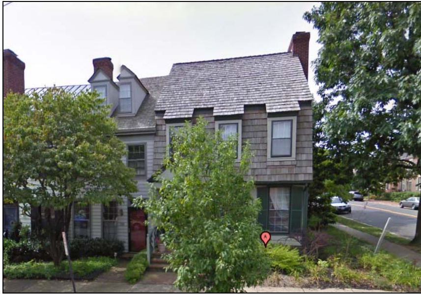
Figure 1: Photograph of Existing Windows – Front Elevation/Gibbon St.
