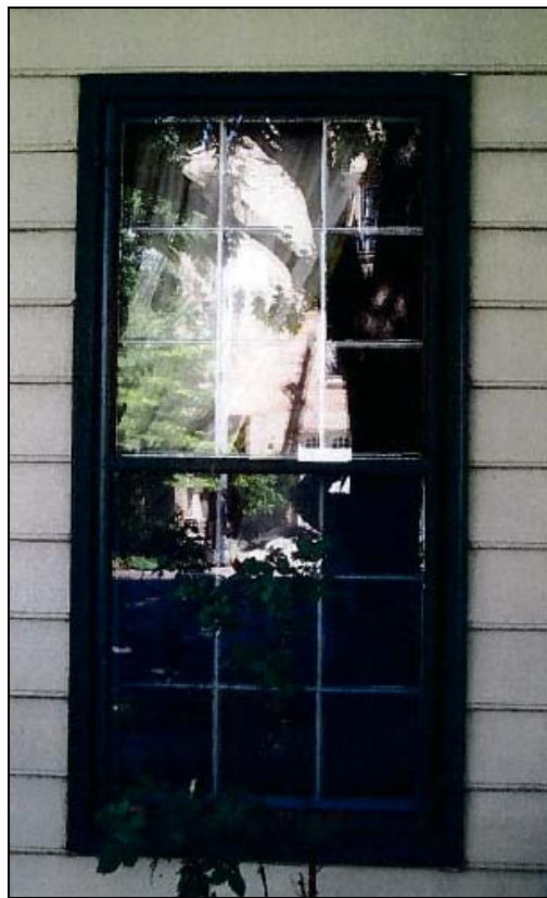
Figure 4: Photograph of Existing Window
