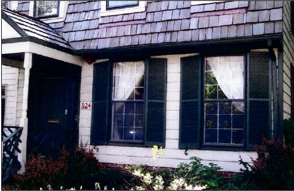
Figure 3: Photograph of Existing Windows
