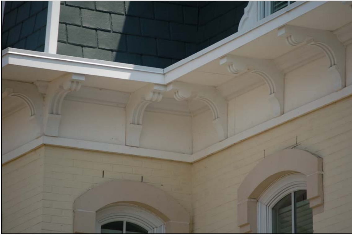
Figure 1. Detail of cornice.
