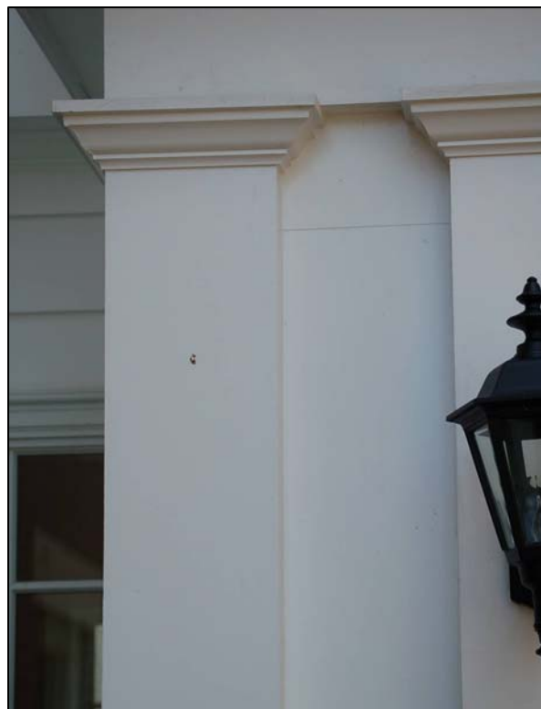
Figure 2. Detail of column.
