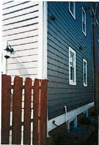
Close up view of siding of 712 from the rear alley
