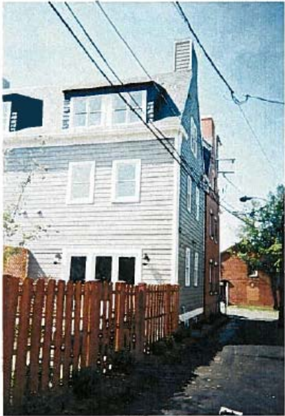
Rear patio door view from the alley of 712
