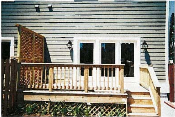
View of patio doors of 712 Wythe Street
