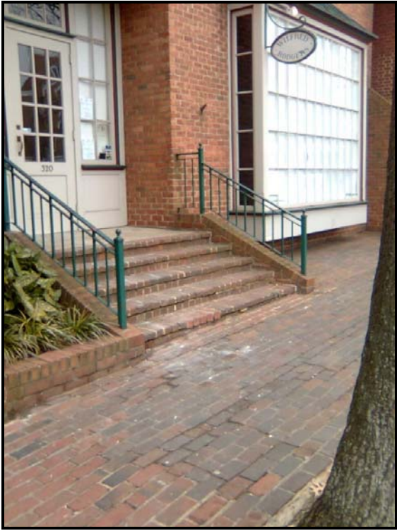
Figure 2: View of Existing Stoop looking West on King Street
