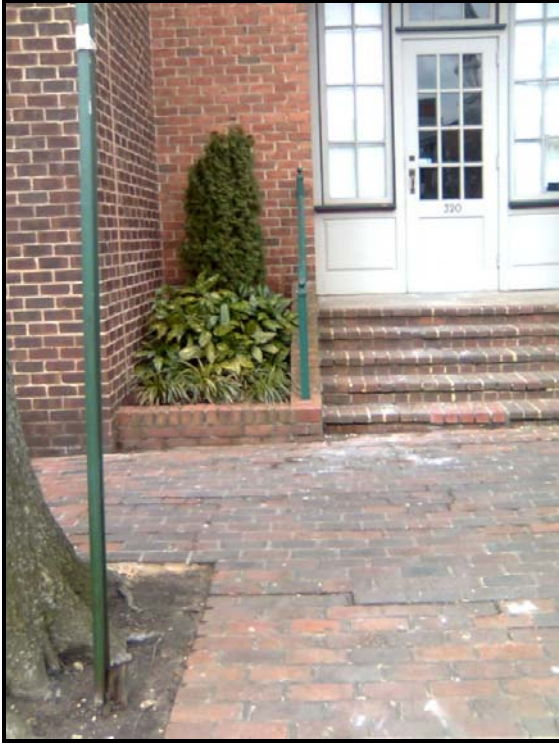
Figure 3: View of Stoop looking South
