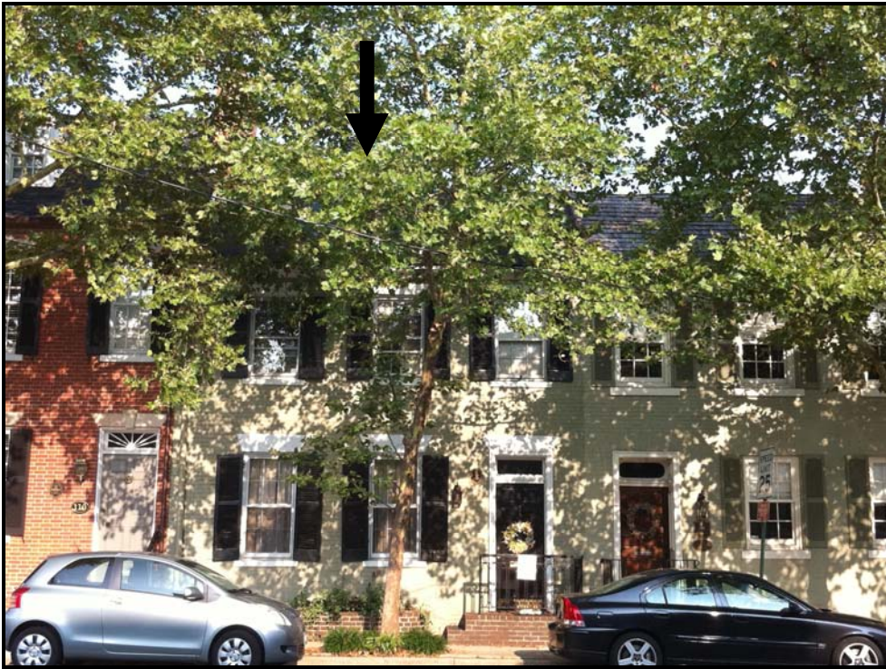
Figure 1. Front facade of 112 N Patrick St.
