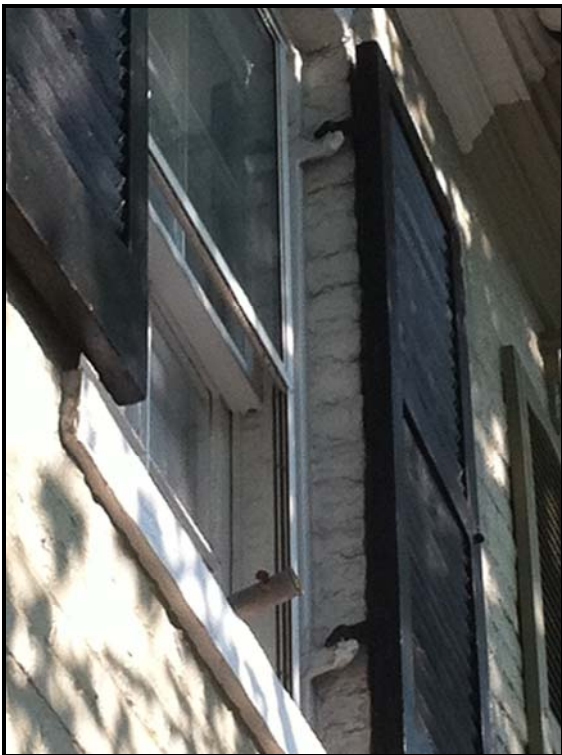
Figure 2. Detail of existing replacement window.
