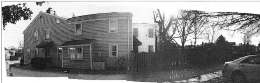
Figure 2: Existing rear elevation
