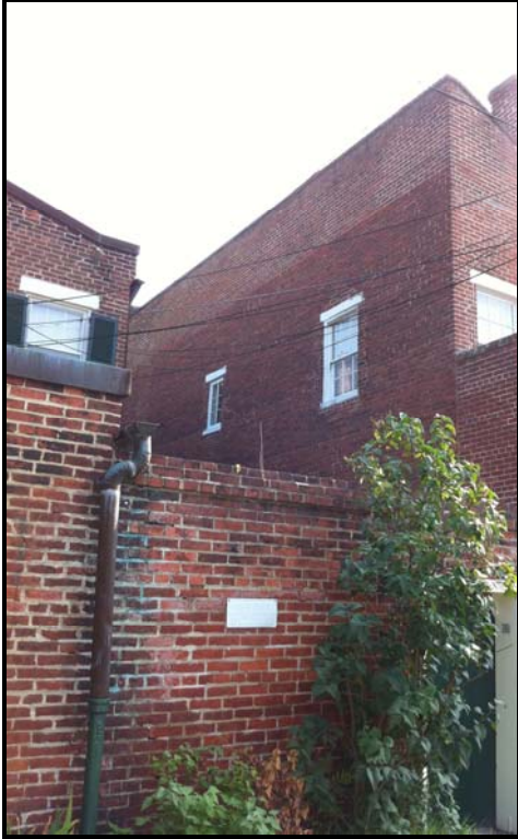
Figure 5. Photograph of west elevation.
