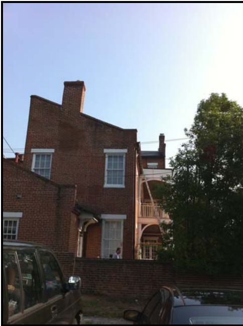
Figure 4. Photograph of rear elevation.
