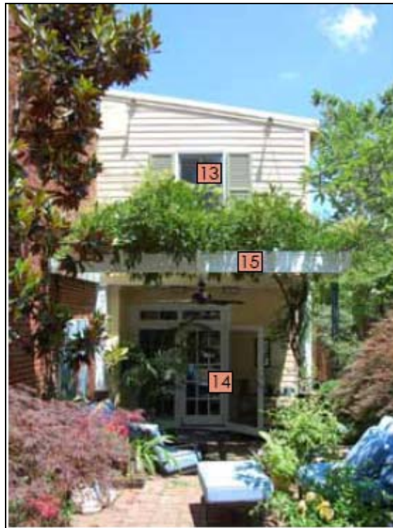
Figure 3. Existing south (rear) elevation.
