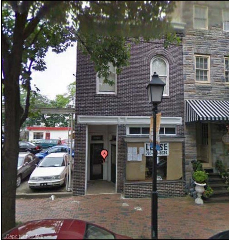
Figure 1. Front elevation of 1314 King Street.
