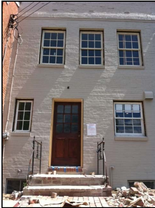
Figure 1. Front elevation with original windows with trim already removed.
