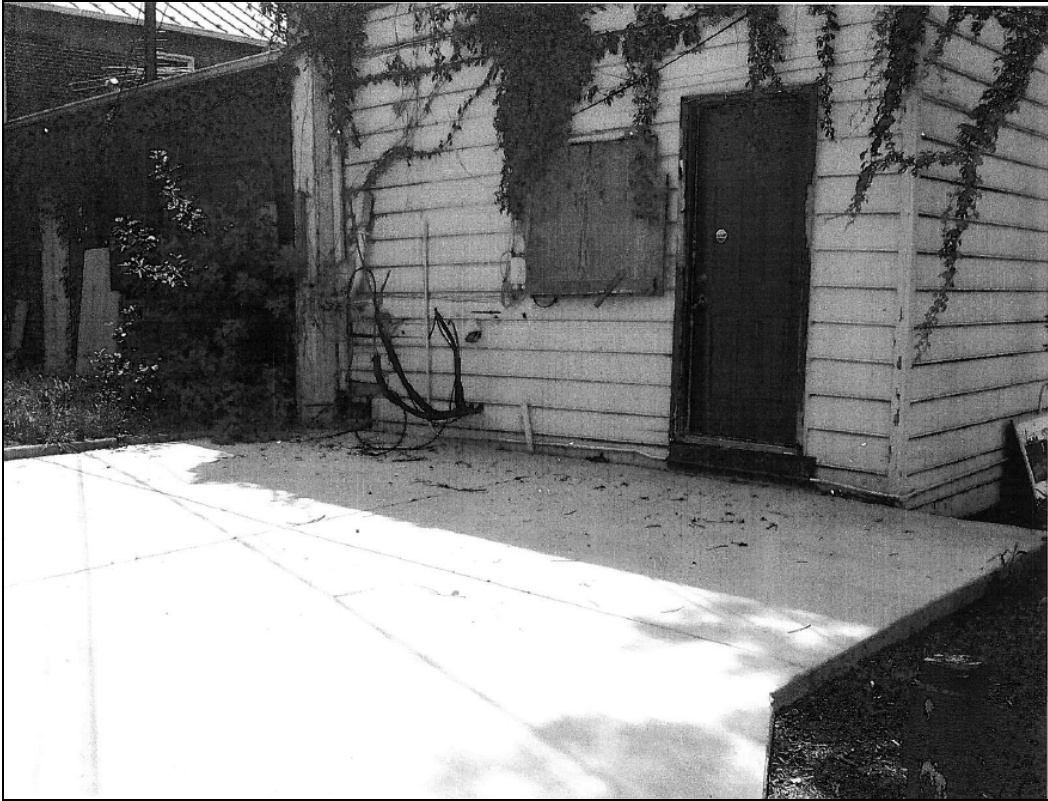
Figure 3. Existing conditions at rear elevation.
