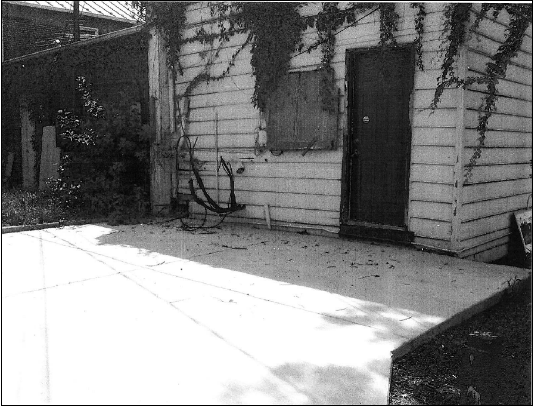
Figure 3. Existing conditions at rear elevation.
