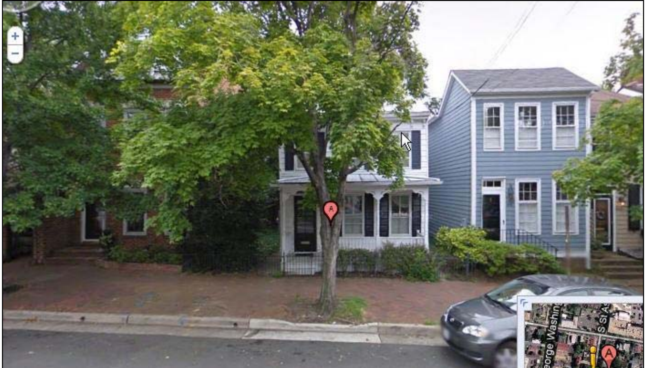
Figure 4. Front (west) elevation of 620 South Saint Asaph with adjacent properties (Source: Google Streetview).
