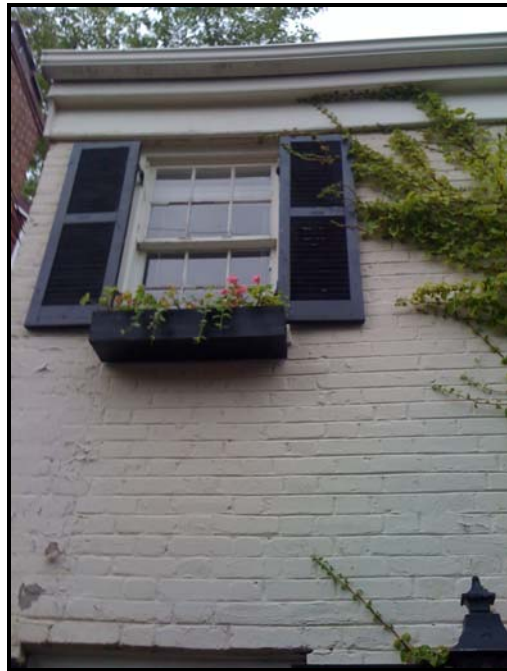
Figure 4. Second Floor Window - Left
