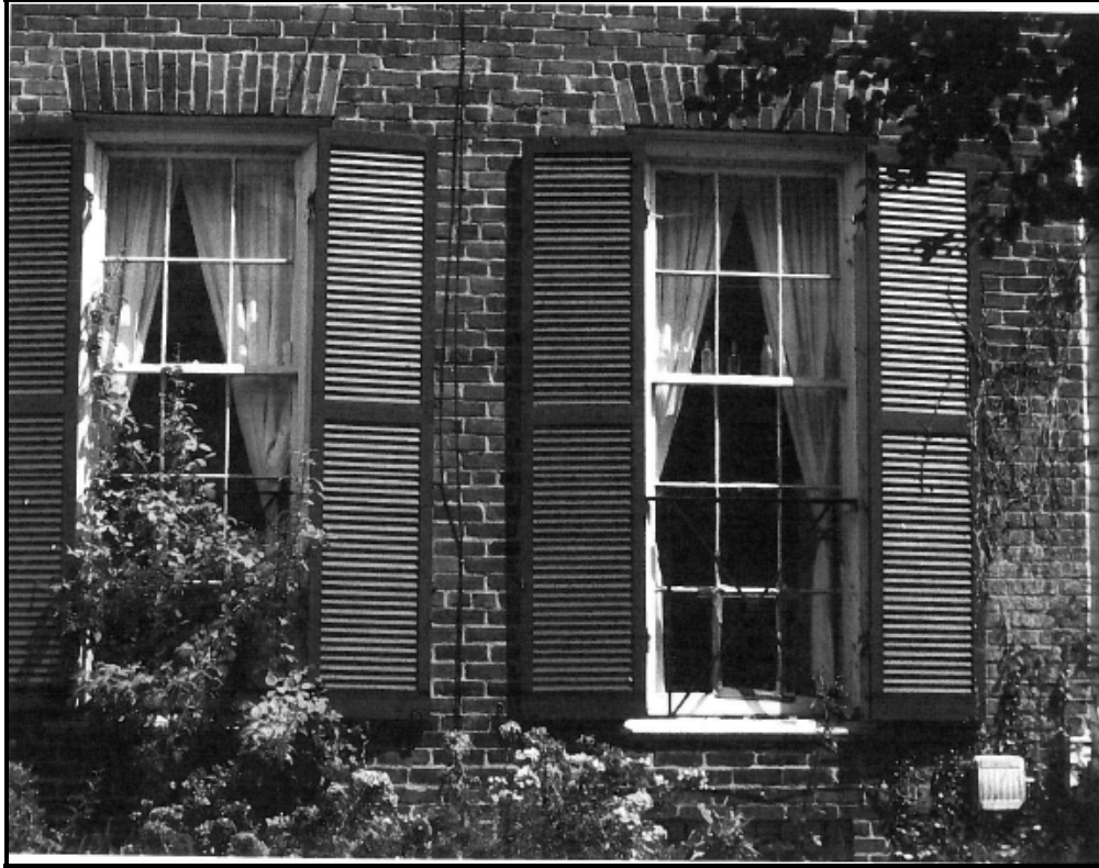
Figure 3: Photo of two first floor windows to be replaced.
