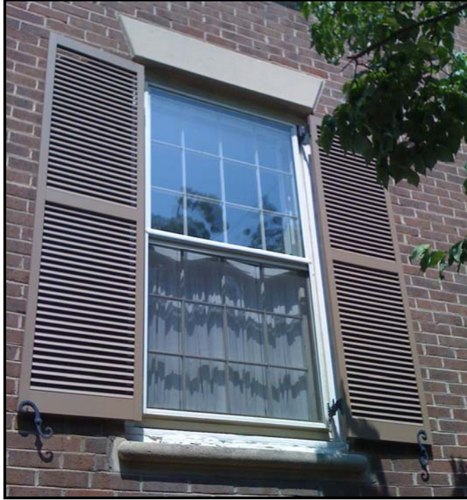
Figure 2. Courtyard Second Floor Window
