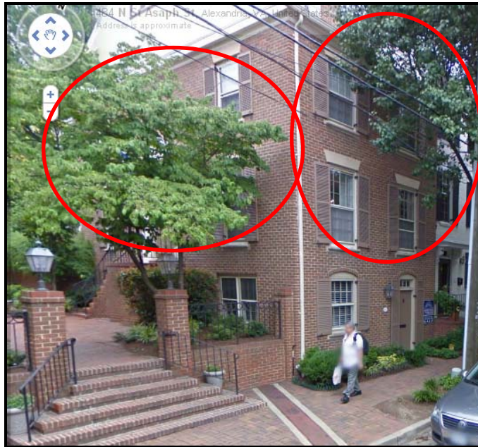
Figure 1. View from Right of Way
