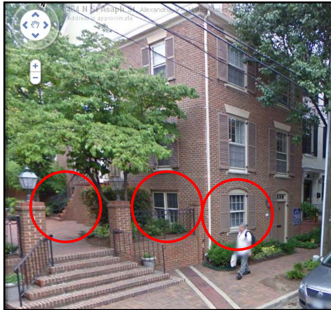
Figure 1. View from Right of Way
