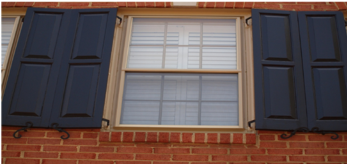
Figure 2. Existing windows, rear (east) elevation.
