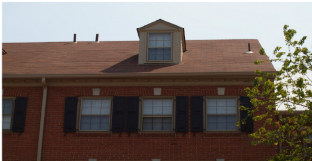
Figure 1. Existing windows, front (west) elevation.
