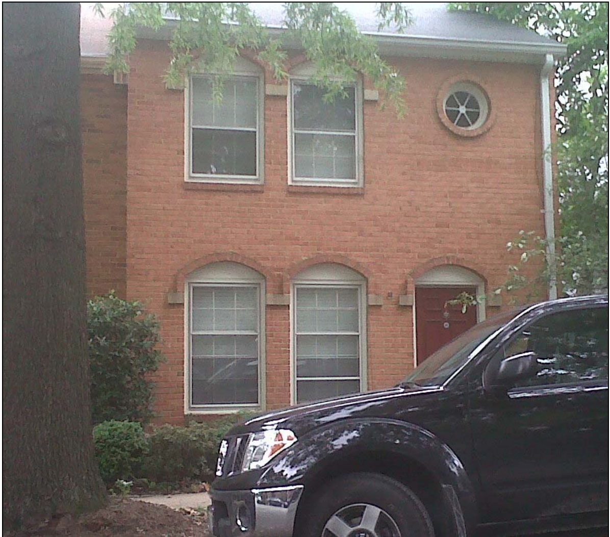
Figure 1. Existing windows, front (east) elevation.
