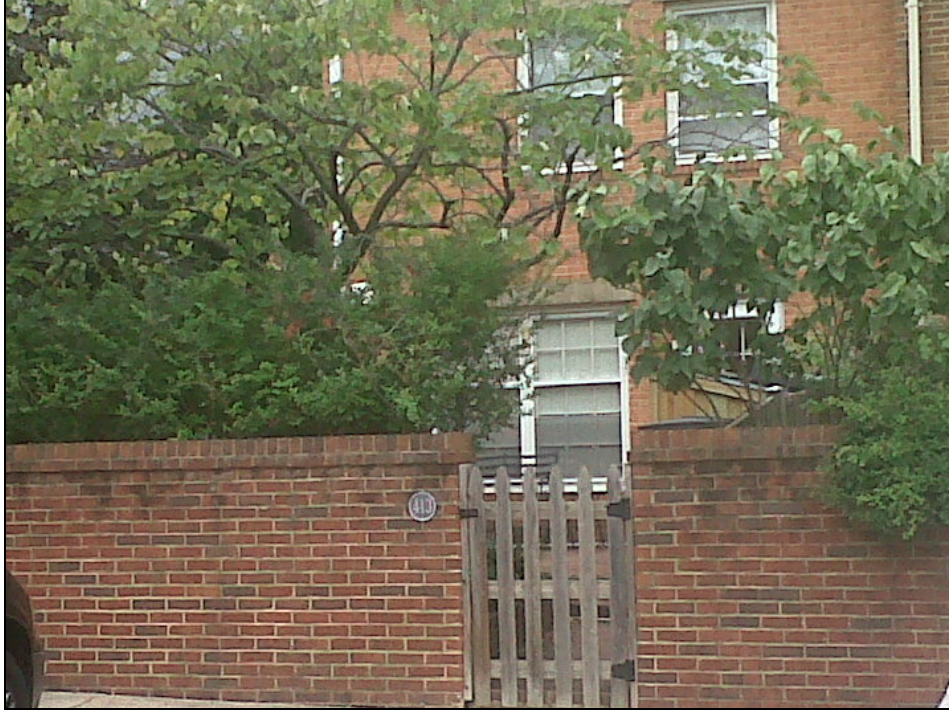
Figure 2. Existing windows, rear (west) elevation.
