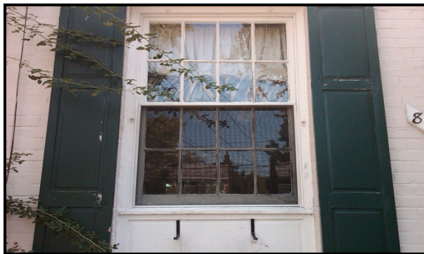
Figure 2: Existing first floor window.
