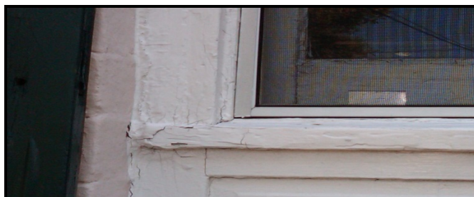
Figure 3: Existing window framing.
