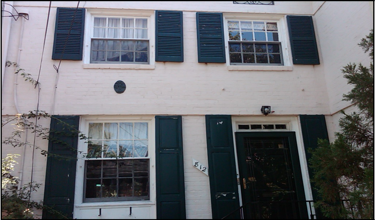
Figure 1. Photo of front façade of 812 South Royal Street
