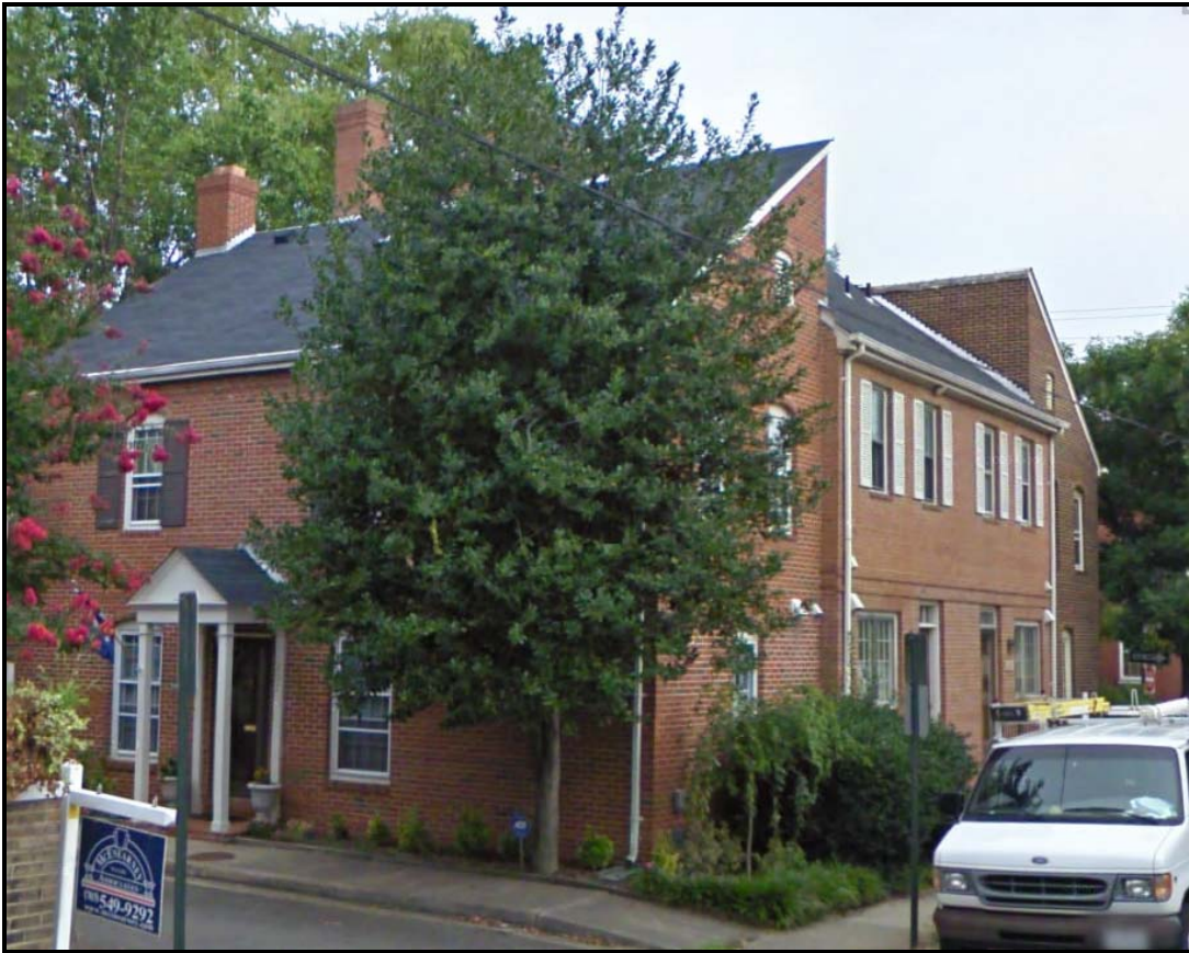
Figure 1. View of Subject Property
