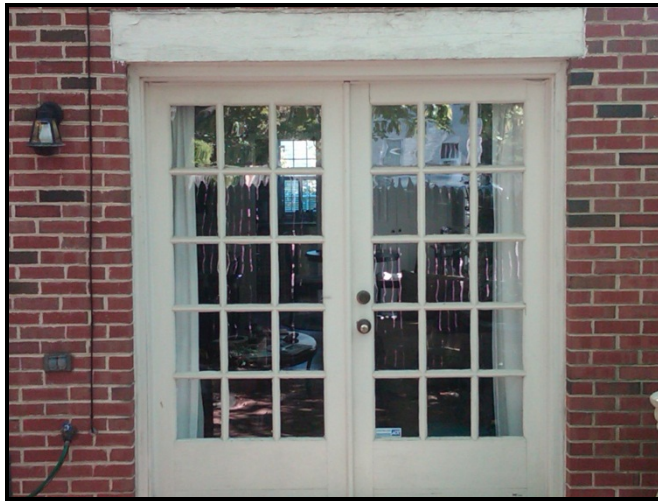
Figure 6. Existing Doors – Rear Elevation
