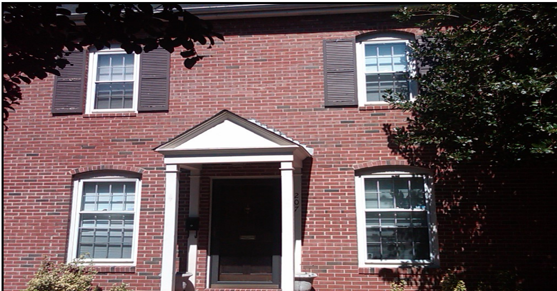
Figure 2. Existing Windows - Front Elevation
