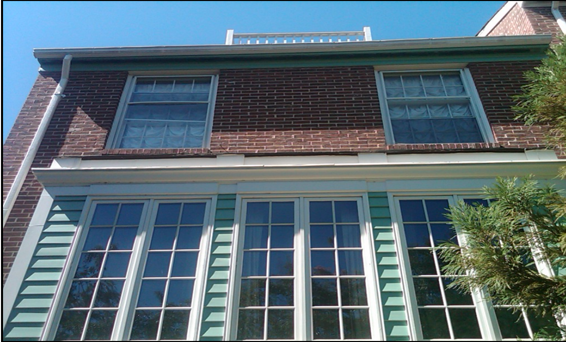
Figure 3. Existing windows - rear elevation
