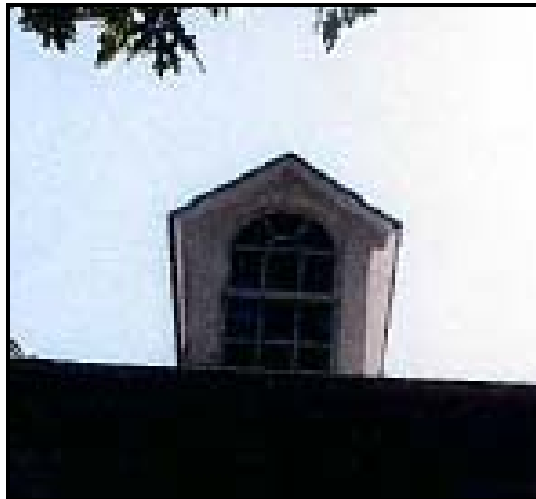
Figure 4. Detail of Existing Window
