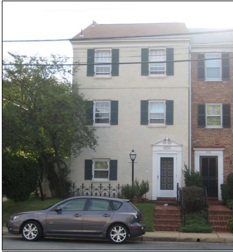
Figure 1. Front (west) elevation of 600 South Royal Street.
