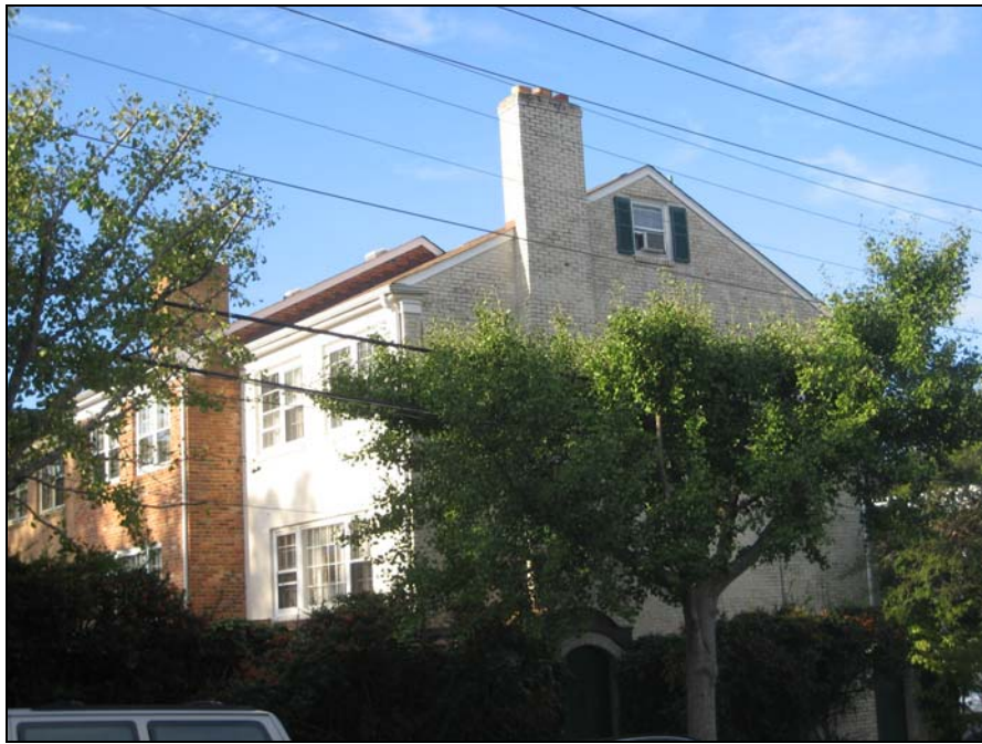
Figure 2. Rear (east) and side (north) elevation.
