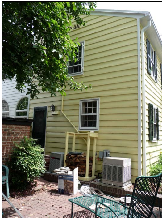
Figure 2. Existing rear elevation - second story is area proposed for demolition.
