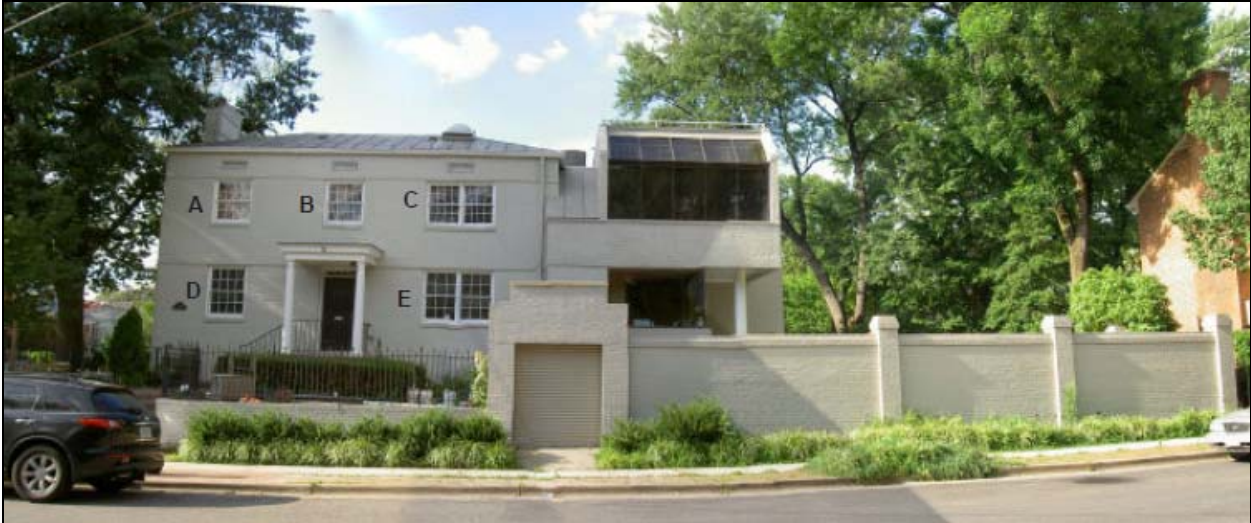
Figure 1. Existing Conditions: Front (south) elevation of 333 Green Street
