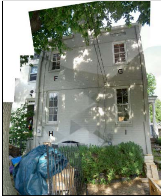
Figure 3. Existing Conditions: Side (west) elevation of 333 Green Street
