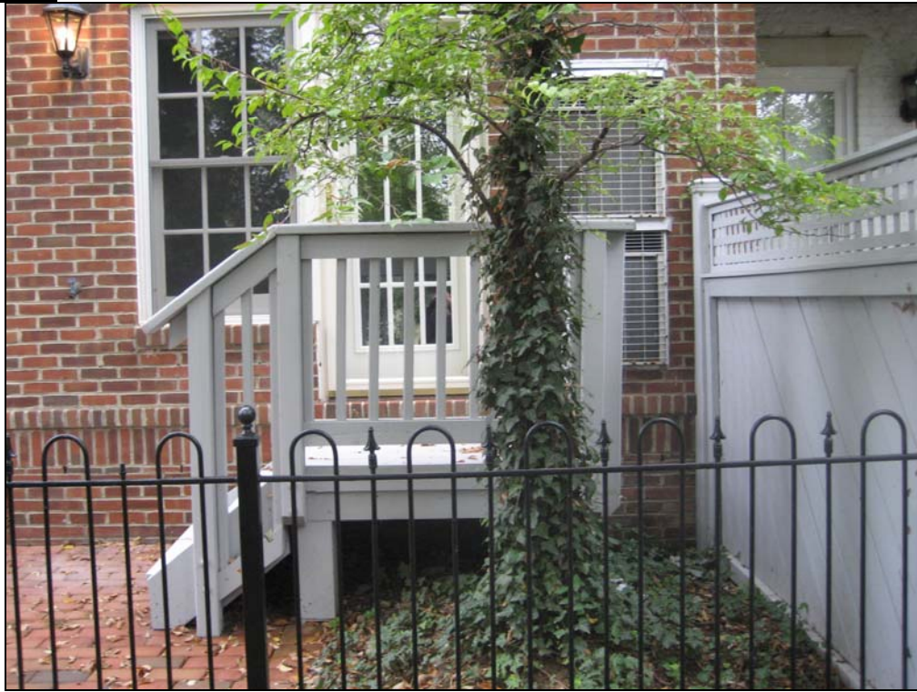
Figure 1. Example of existing wood stoop and railing and through-wall HVAC units.
