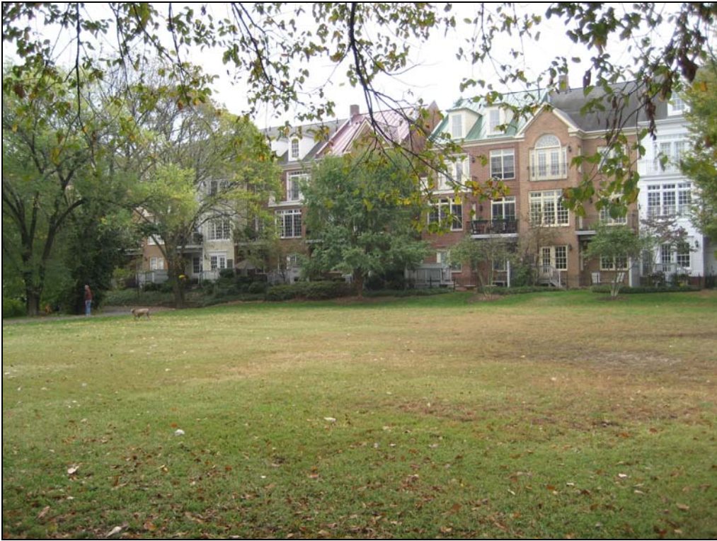
Figure 5. View of rear elevations of Keith's Lane townhouses from park.
