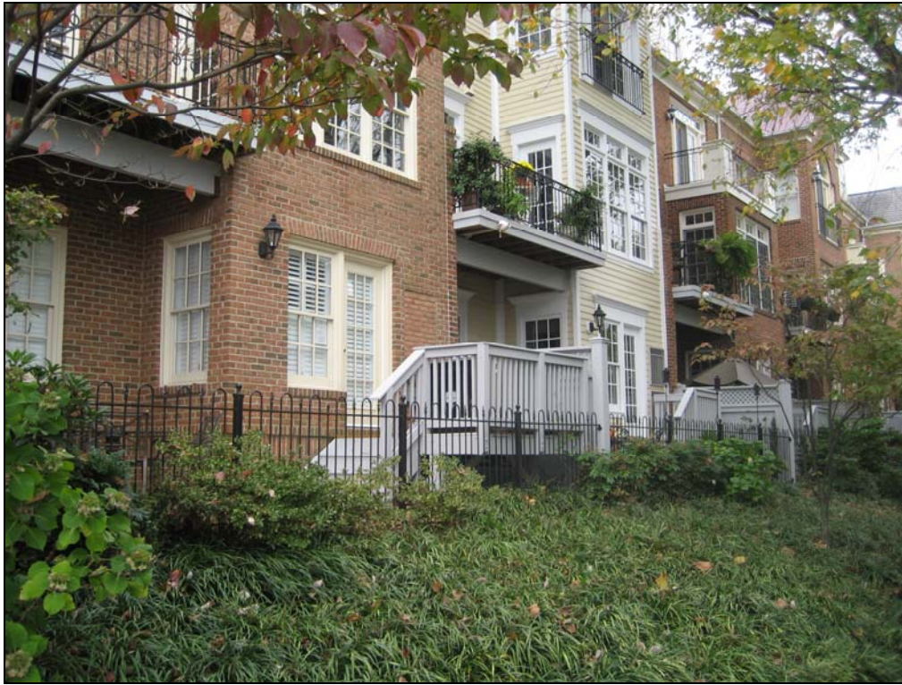
Figure 3. View from park of 9 Keith's Lane with expanded deck and infill brick, and the existing deck configuration to the right.
