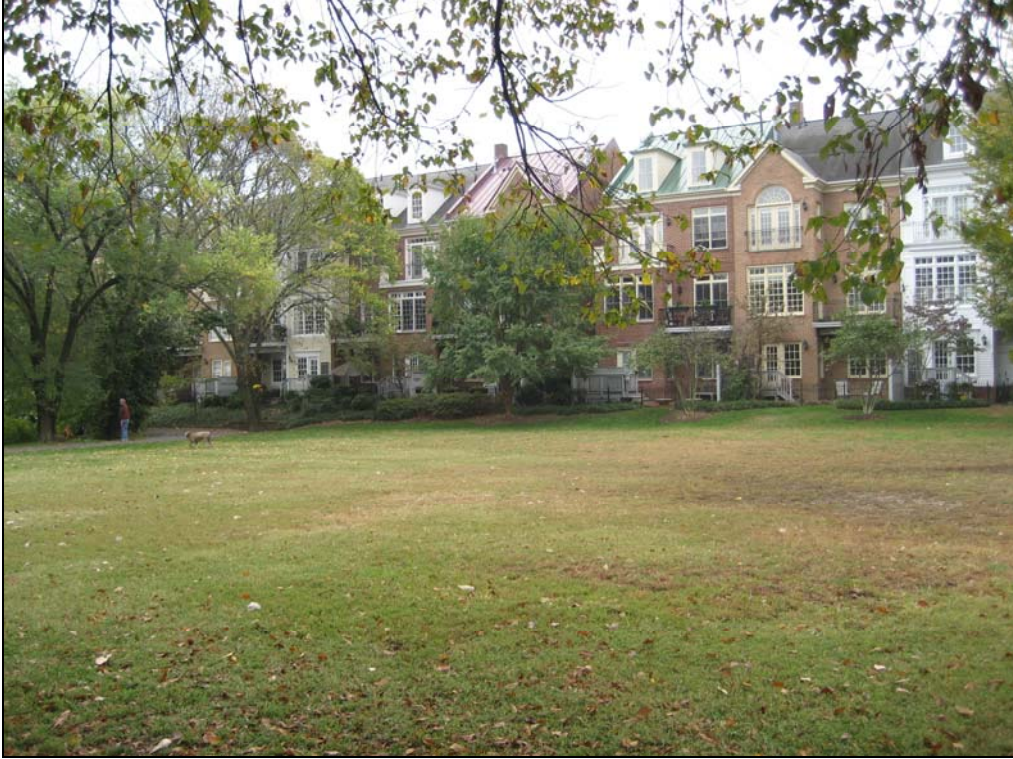
Figure 4. View of rear elevations of Keith's Lane townhouses from park.
