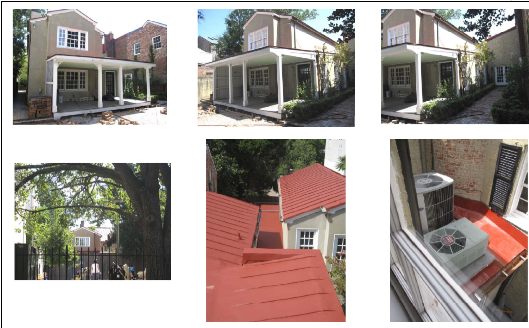
Figure 3. Photos showing existing conditions, location of proposed rooftop mechanical equipment screen wall, view from South Royal Street, and existing HVAC units. The photo in the lower left shows that the first floor porch columns are not visible from South Royal Street or the park.
