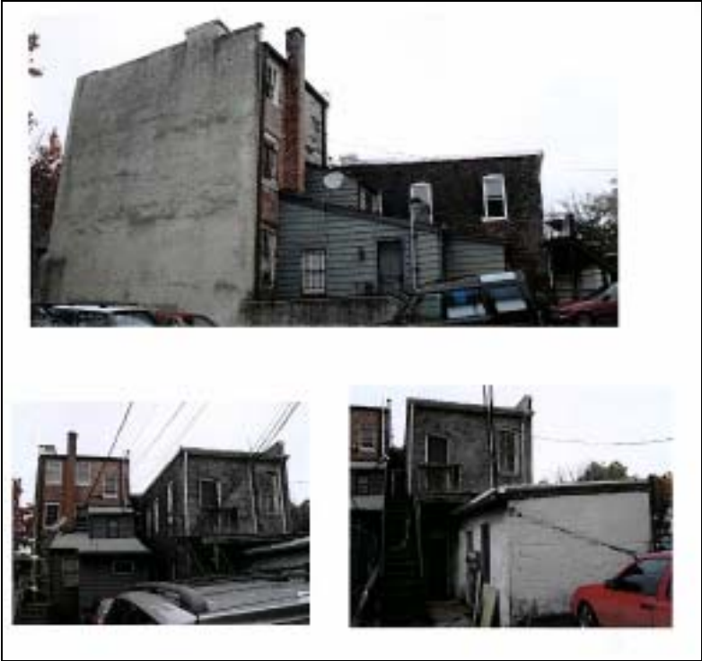
Figure 2. Rear and Side Elevations
