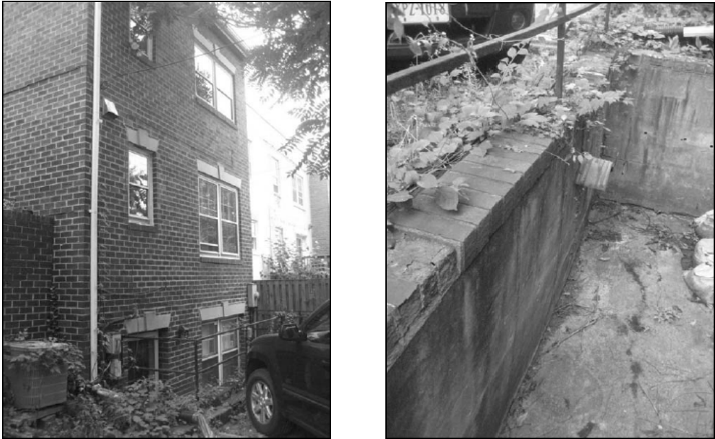
Figure 3. Existing Conditions – Rear Elevation & Areaway
