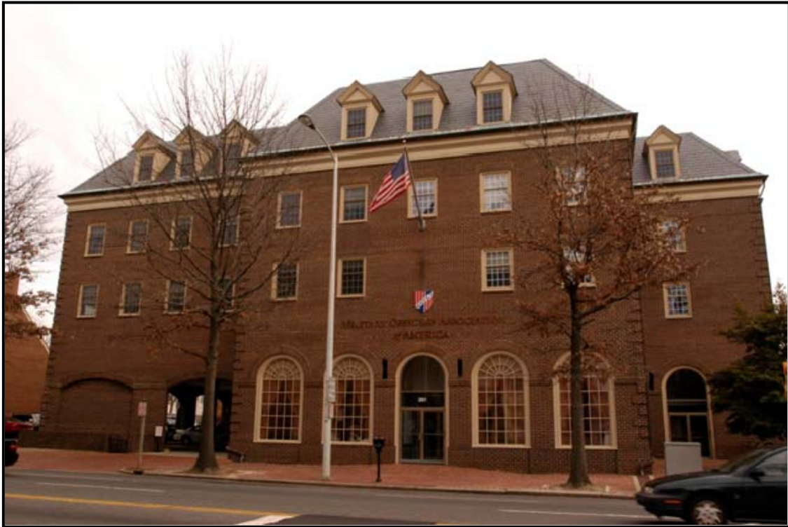
Figure 1: Photo of 201 North Washington Street showing proposed location of light fixtures.
