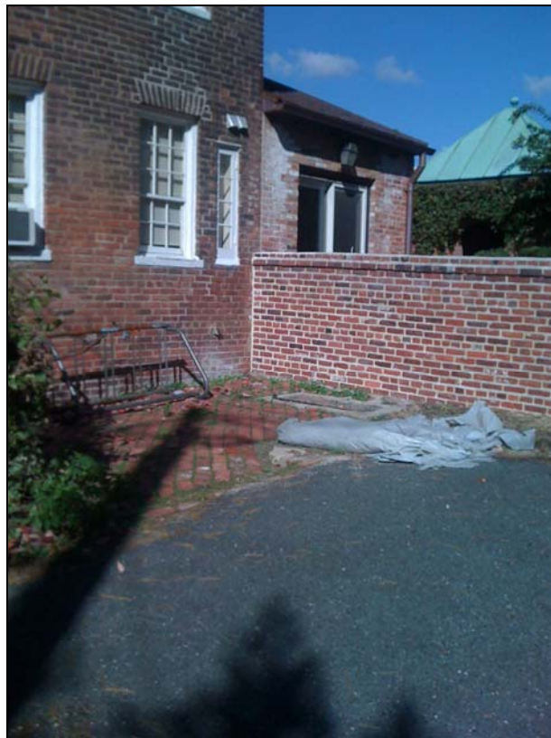
Figure 4. General location (on brick) of HVAC condenser units and screening.
