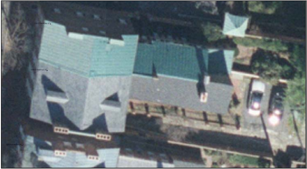
Figure 1. Ariel view of site with existing conditions.
