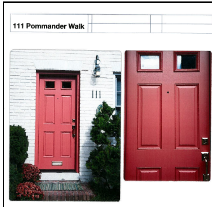
Figure 1: Fiberglass door at 111 Pommander Walk Street
