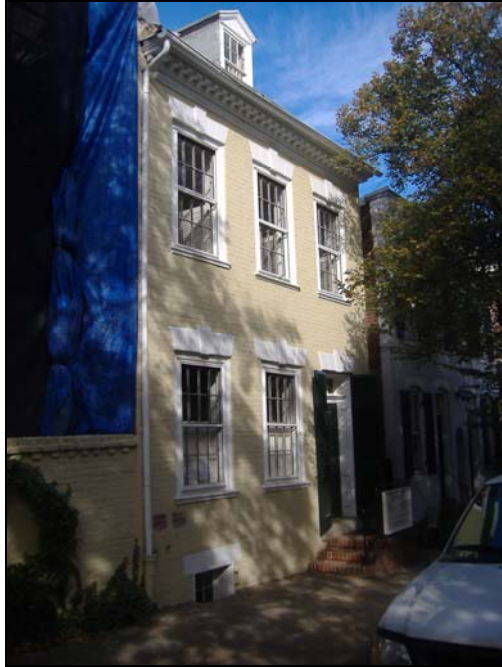
Figure 1. Front (east) elevation.
