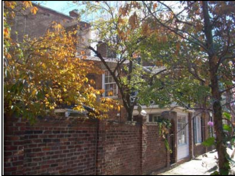
Figure 7: Views of existing covered porch from South Alfred Street
