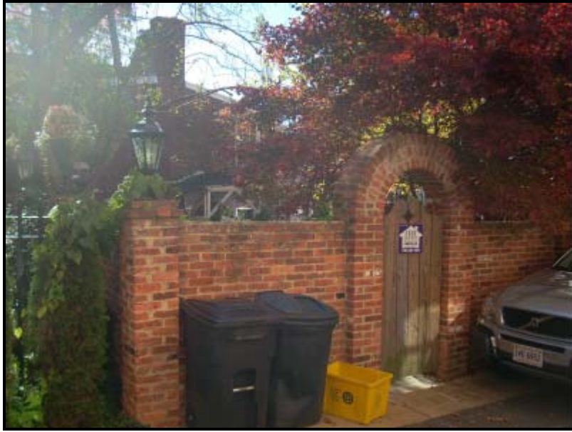
Figure 9: Views of existing covered porch from adjacent alley
