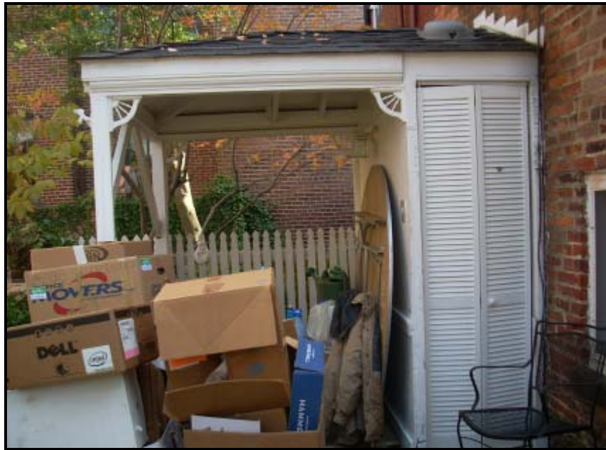
Figure 10: View of existing covered porch from inside brick perimeter wall
