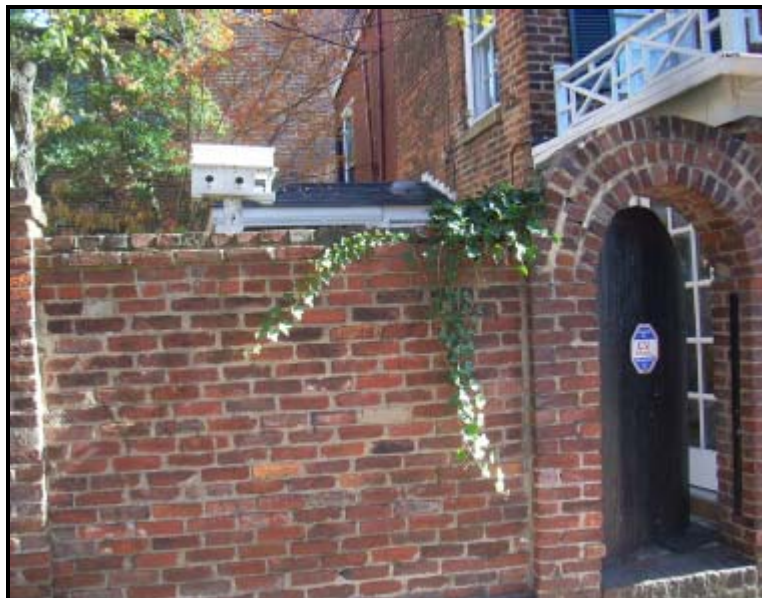
Figure 8: Views of existing covered porch from South Alfred Street
