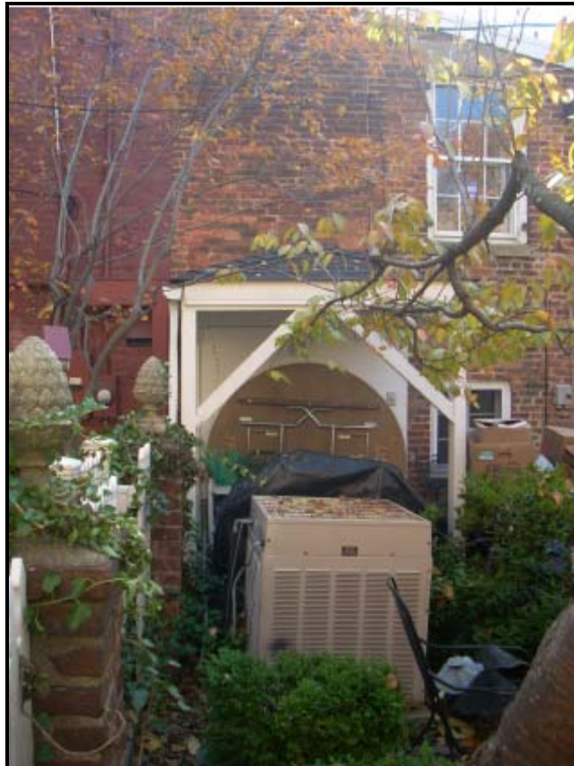
Figure 12: View of existing covered porch from inside brick perimeter wall
