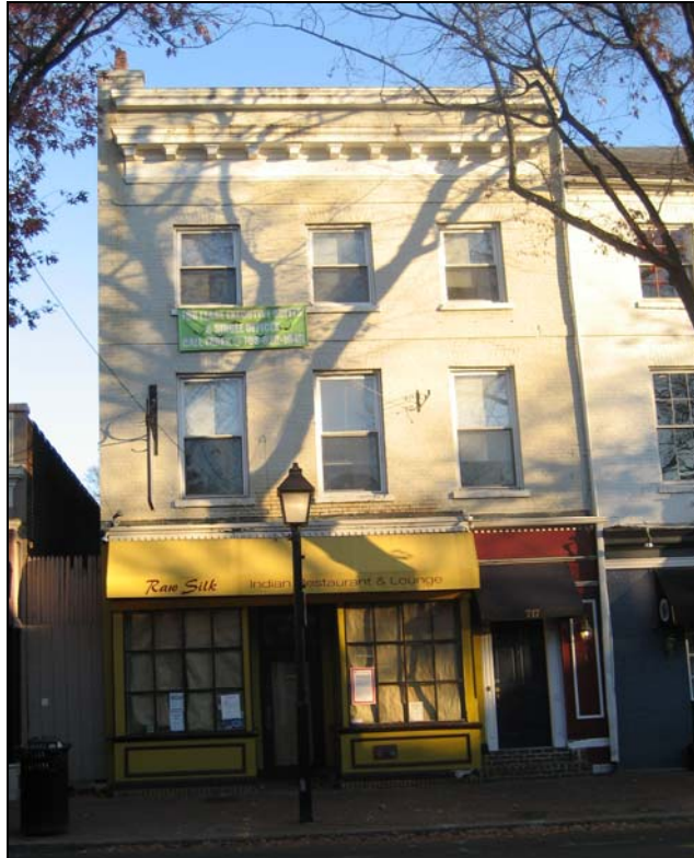
Figure 1. Existing front (south) elevation
