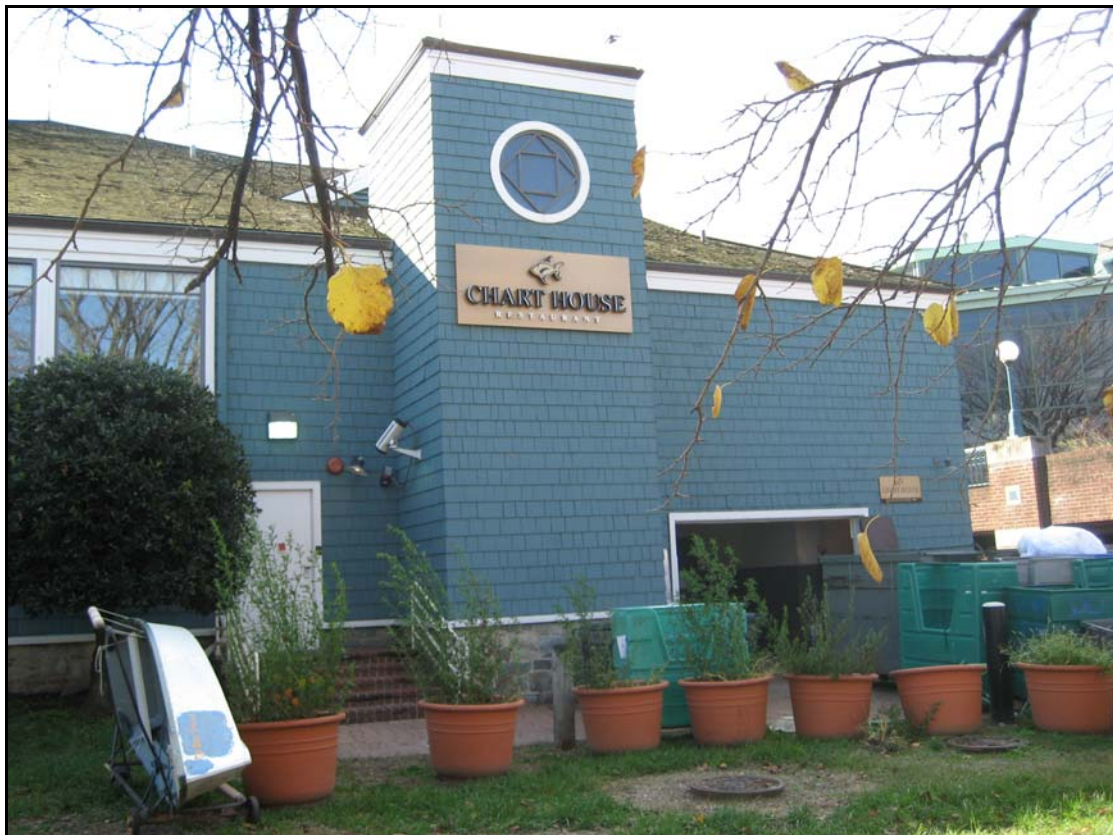
Figure 2. Existing conditions, looking southwest.
