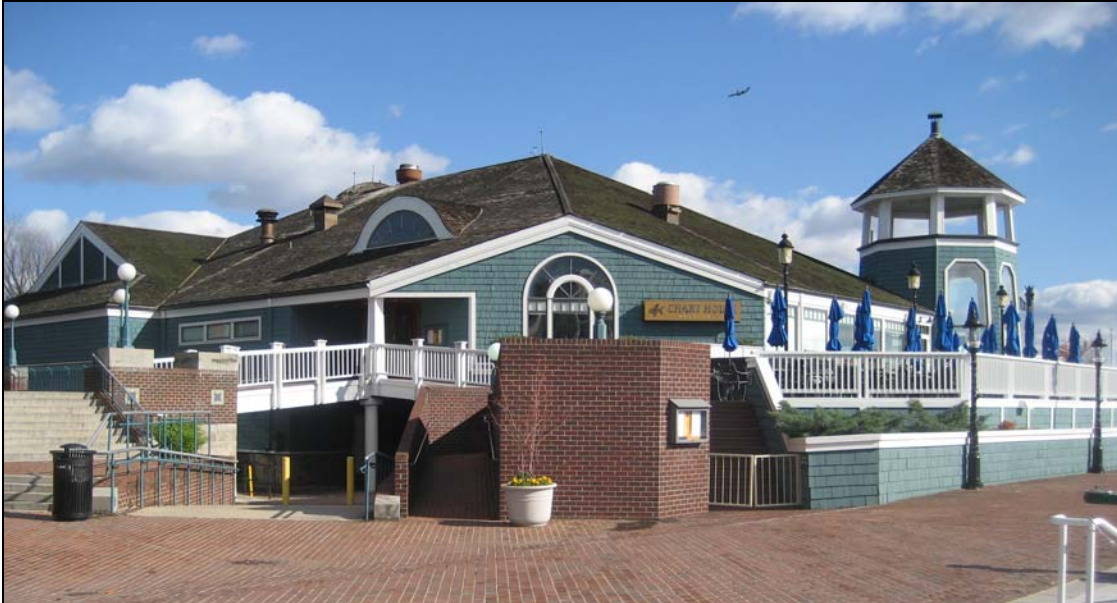
Figure 1. Existing conditions, looking northeast.
