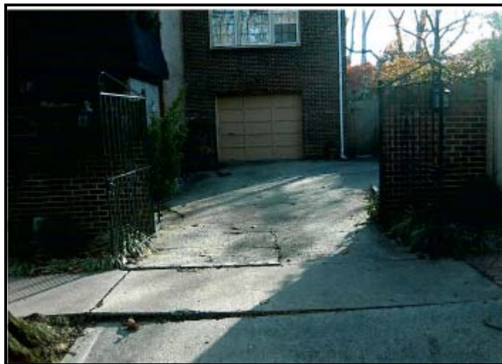
Figure10: 328 North Pitt Street metal gates.
