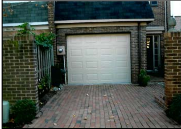
Figure 5: 340 North Pitt Street rear entrance (no gates).
