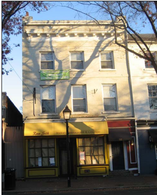
Figure 1. Existing front (south) elevation
