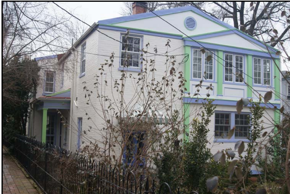
Figure 5: North (rear) elevation.
