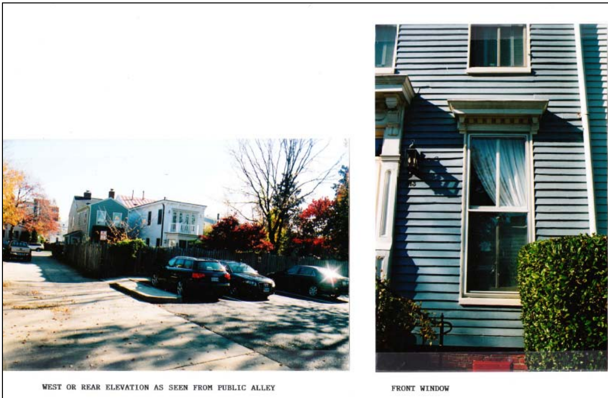
Figure 2. West (rear) elevation from public alley (not visible, third house in) and front window.
