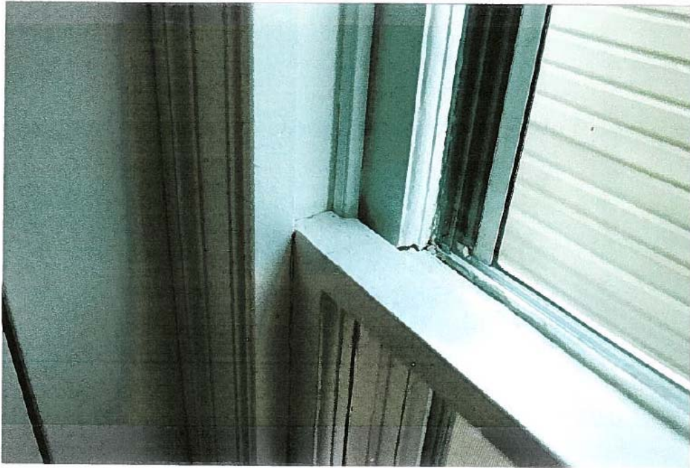
INTERIOR VIEW OF WINDOW SASH AT JAMB
