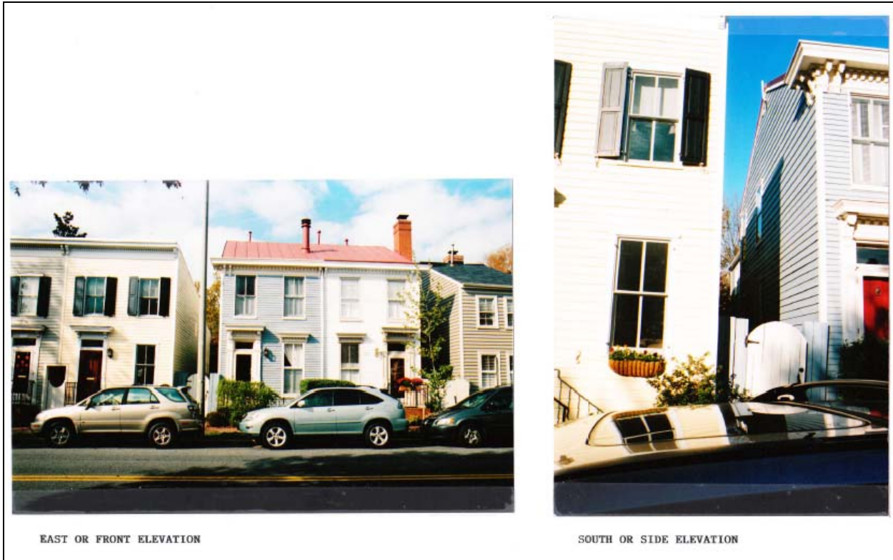
Figure 1. East (front) elevation and south (side) elevation.
