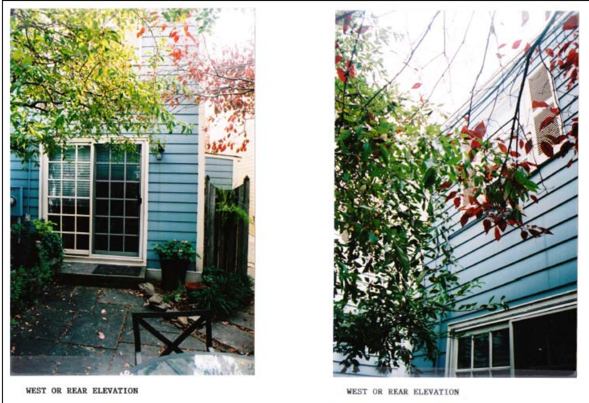
Figure 3. West (rear) elevation with sliding glass door to be replaced view of area for new shed (behind wood fence).
