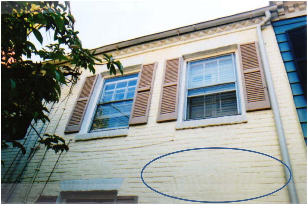
Figure 4: Detail of jack arch above entry
