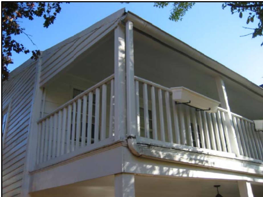
Figure 2: Existing Open Porch
