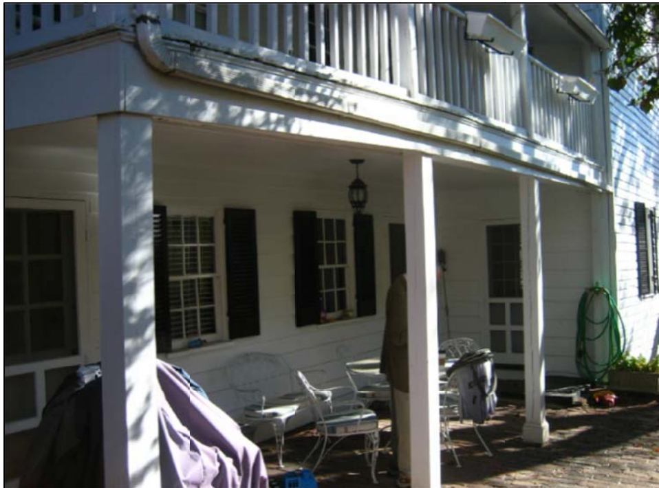
Figure 4: Existing Open Porch
