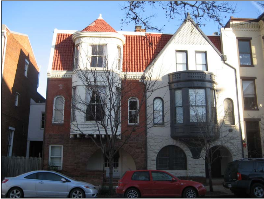
Figure 1. Front elevation of 917 Prince Street (on left) with turret with existing clay tile roof.
