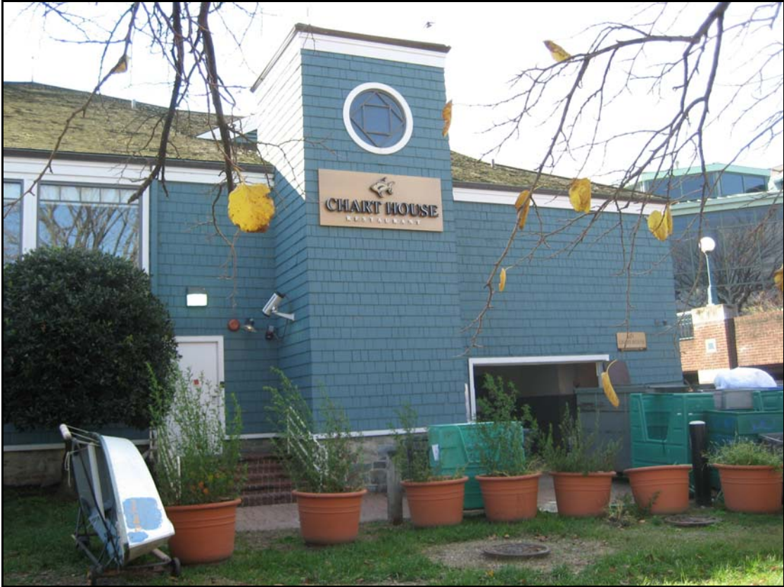
Figure 3. Existing conditions, looking southwest.
