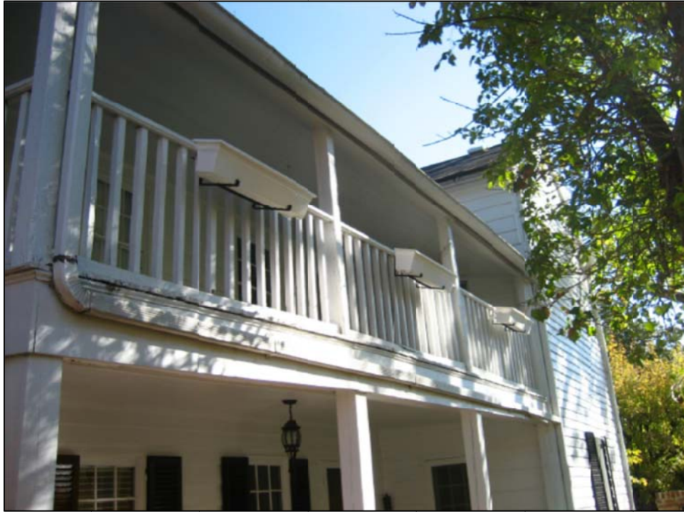
Figure 3: Existing Open Porch
