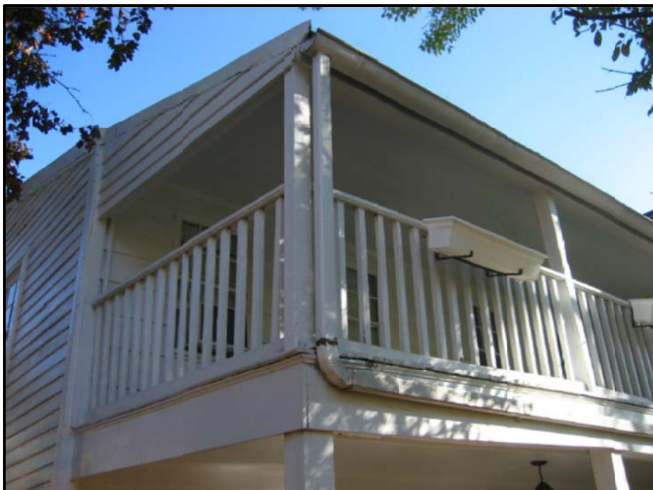
Figure 2: Existing Open Porch
