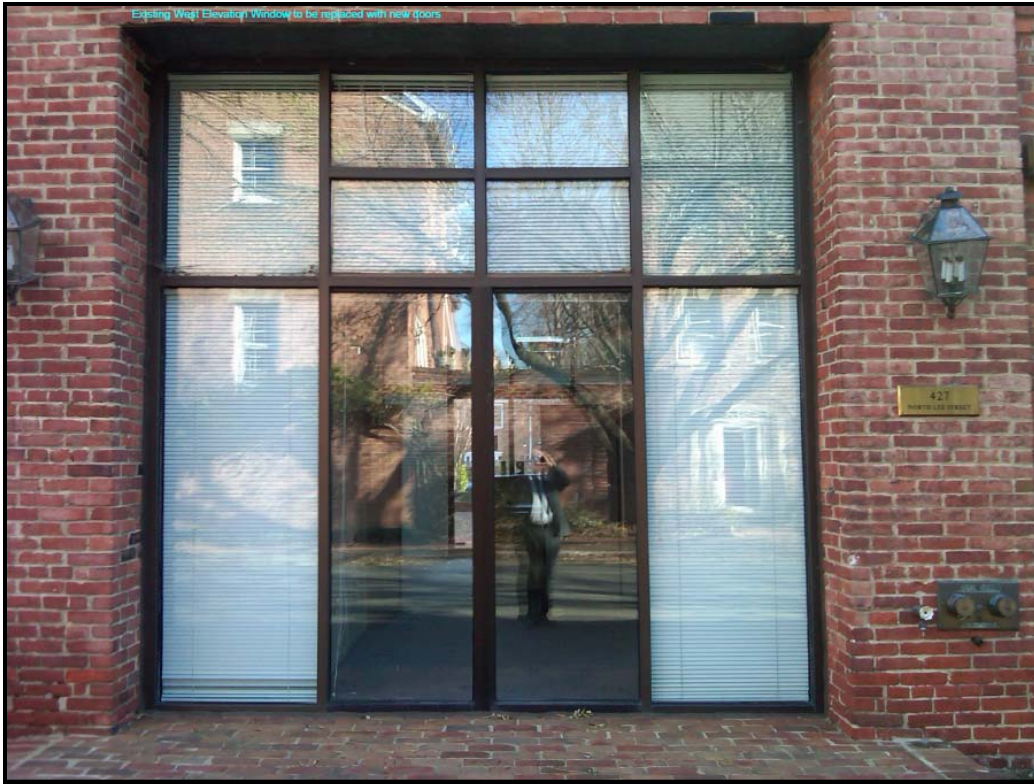
Figure 3. Photo of existing west (North Lee Street) elevation.
