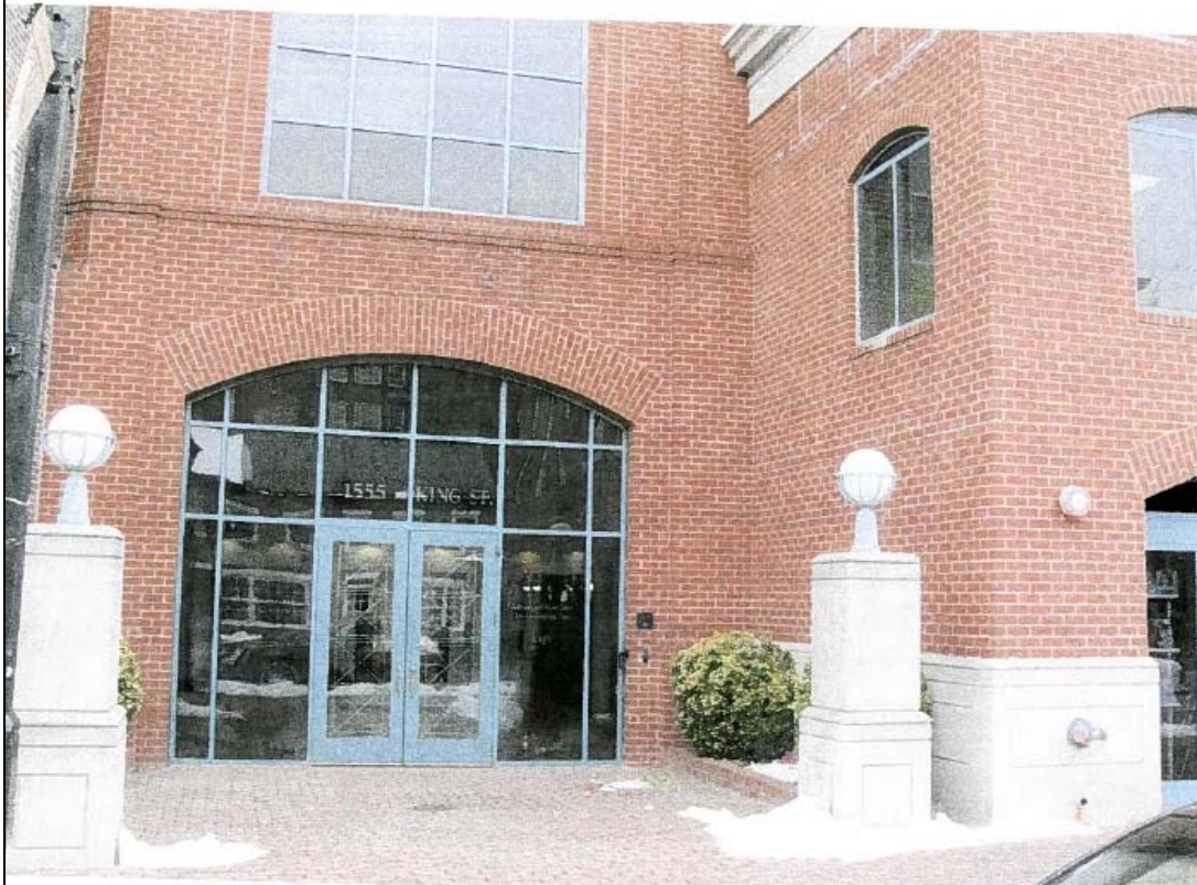
Figure 1. View to rear from alley, above, and front (south) elevation, below.
