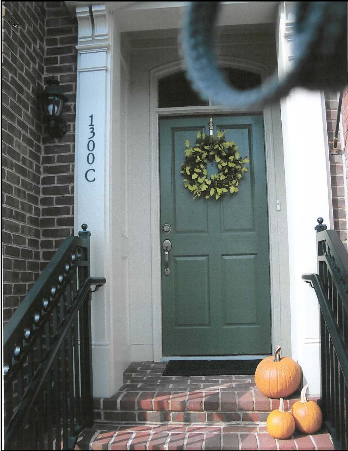
Figure 1. Photo of Existing Front Door
